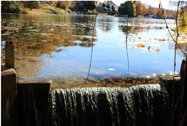
1. Inlet of weir structure in Barnes Lake
