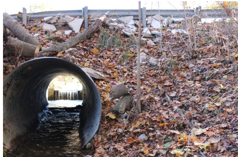
12. Looking at downstream slope of road
