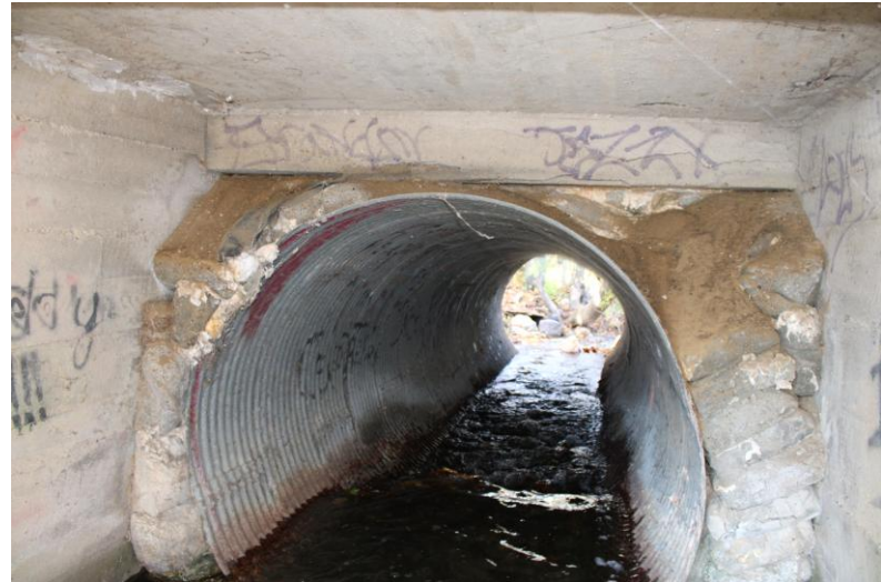
4. Where concrete structure connects to corrugated metal pipe (CMP) in structure
