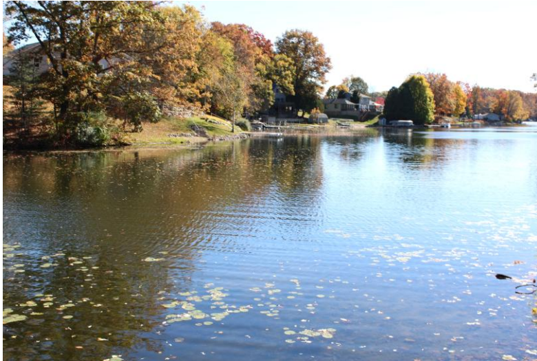
17. Approach channel to structure
