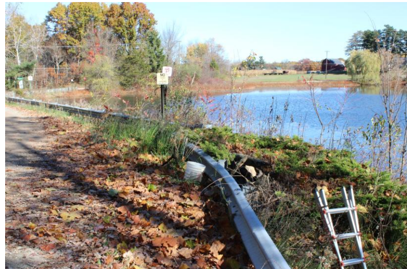
16. East side of roadway, with well established vegetation & shrubs to prevent erosion
