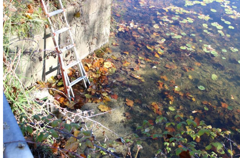
18. Concrete wing wall of structure.
