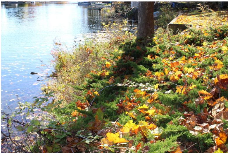
19. Southwestern embankment above steel sheet pile, with well established vegetation for erosion protection.
