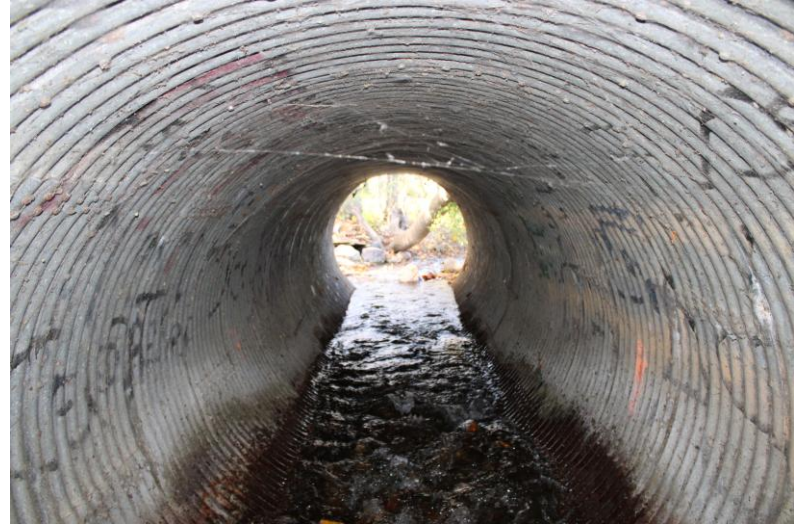
10. Outlet CMP looking downstream.
